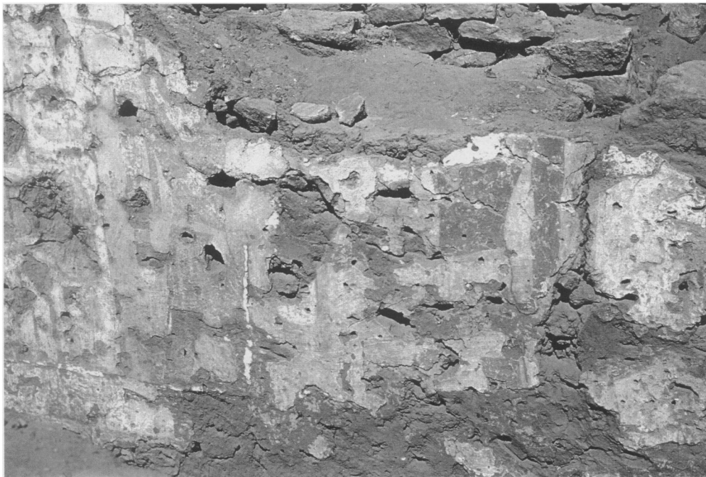
2. The north-west wall of the sanctuary after clearance in 2003.
